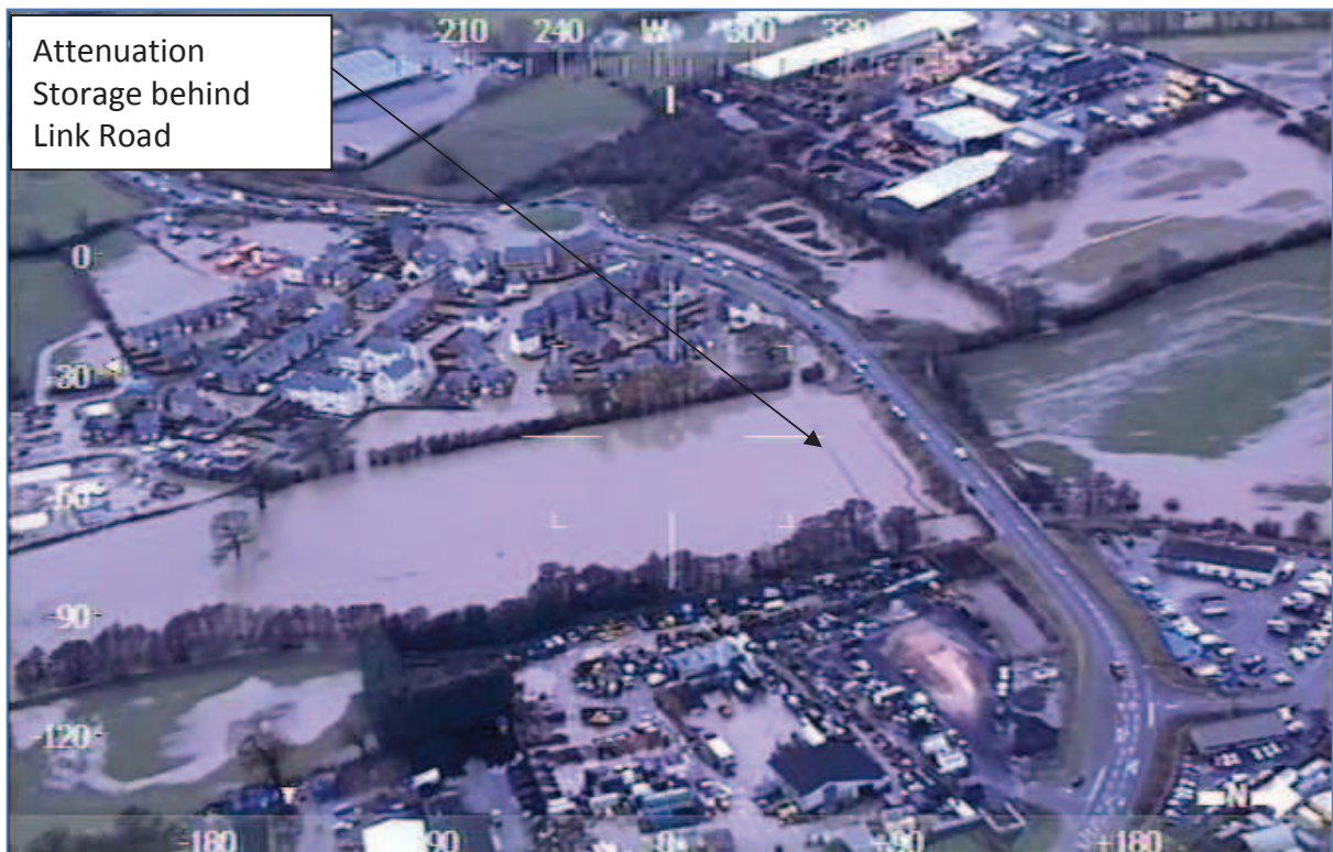
Plate 10 - November 2012 flooding to Glasdir (view from east)
