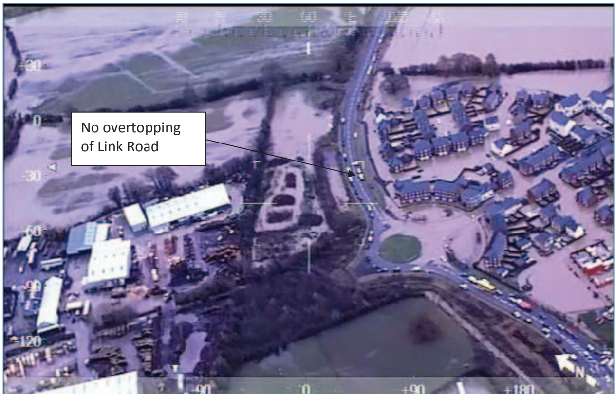
Plate 8 - November 2012 flooding to Glasdir
