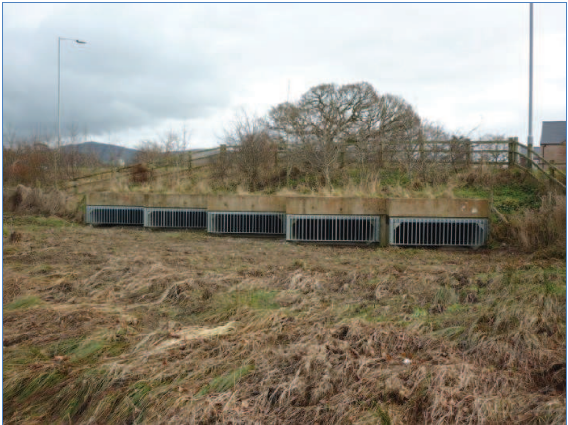
Plate 4 - Ruthin Link Road Culverts
