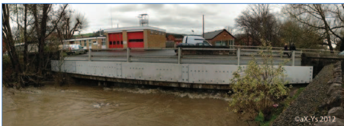
Plate 3 - River Clwyd Bridge (Upstream View during November 2012 event)
